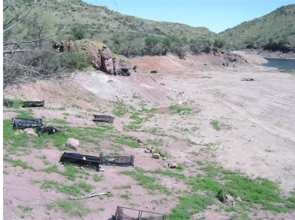
Lake Bottom after Sludge Removal and Fish Habitat Installation
