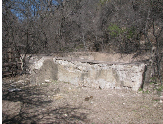
Noonville Building Foundation
