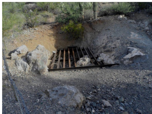
Figure 9. Second Access Shaft
