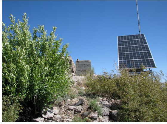
Destroyed Communications Equipment Were Replaced Photo by T. Johnson
