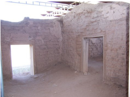
Interior of Main Structure
