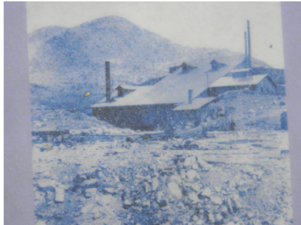
Figure 8. Grand Central Mill
