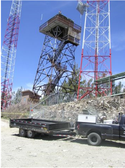
Lookout Cabin Demolition in Progress Photo by T. Johnson
