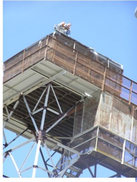
Workman on Roof demolishing the Wood Cabin Photo by Jim Chisholm
