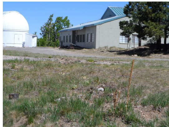
Multi-Purpose Recreation Building Mount Lemmon Air Force Station Photo by T. Johnson
