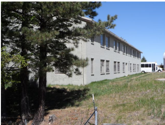
Enlisted Barracks – Mount Lemmon Air Force Station Photo by T. Johnson
