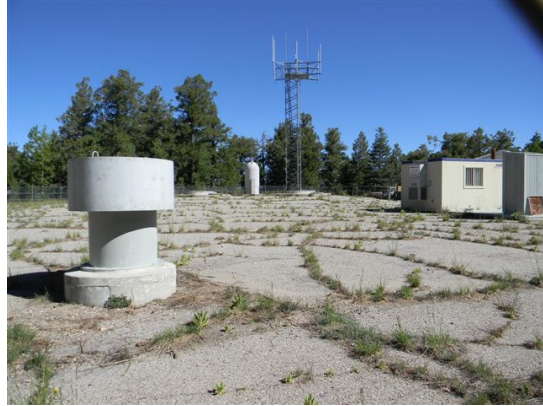
Site of Titan Underground Communications Center Photo by T. Johnson - 2012
