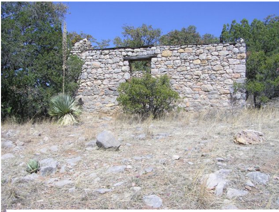
Possible Explosives Storage Building
