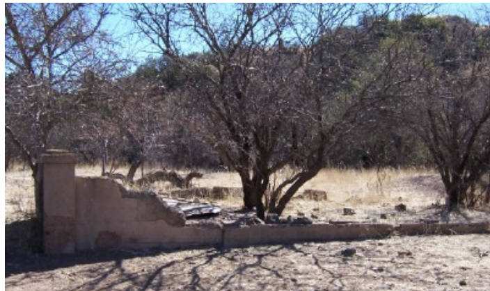
Remains of the Rosemont Ranger Station Photo by T. Johnson
