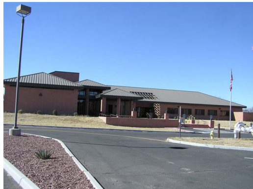
Nogales Ranger Station – 2011 Photo by T. Johnson
