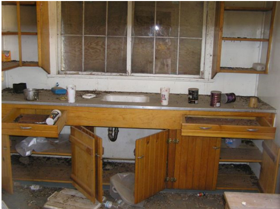
Figure 6. Condition of Kitchen Area
