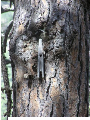
Insulator Arm Mounting
